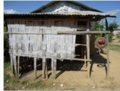
Seilal JB School Kitchen Shed
