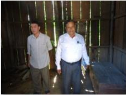
Khumujamba Jr HS Kitchen Shed cum store room
