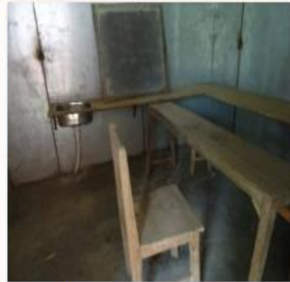
Thoubal Wangmataba Manishang PS kitchen Shed
